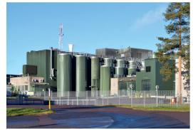
The upper picture: Valio Ltd, Haapavesi production plant From left to right: CIP facilities, Cooling compressor, Raw material silos
